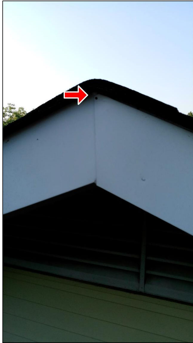
1.0 Item 2(Picture) Missing ridge vent
