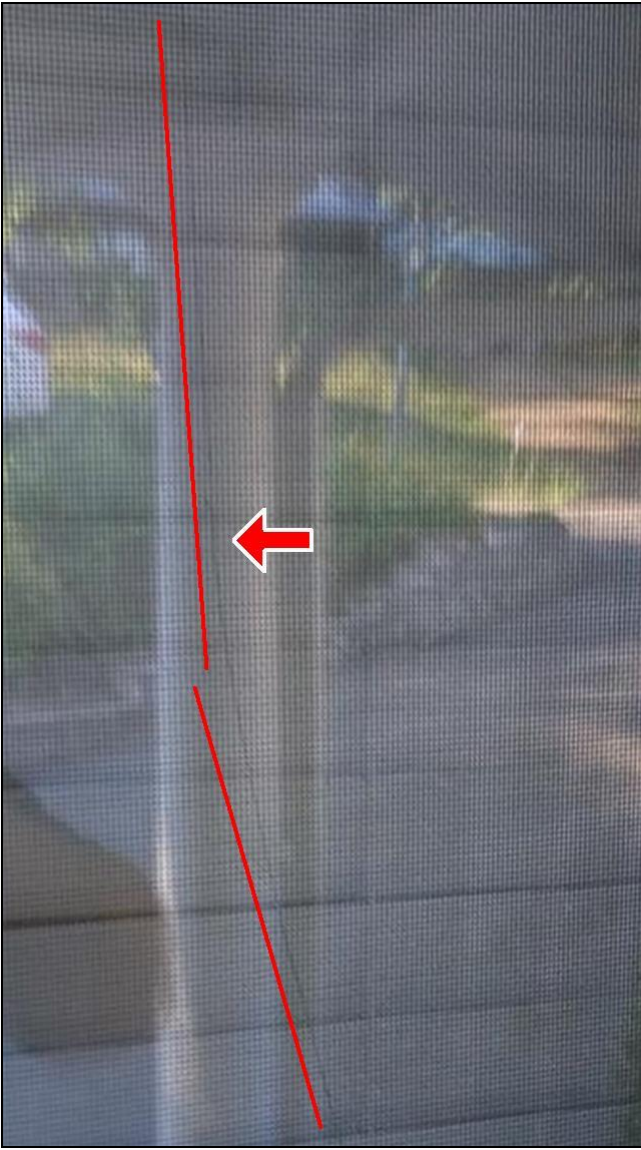
2.2 Item 1(Picture) Cracked front facing window
