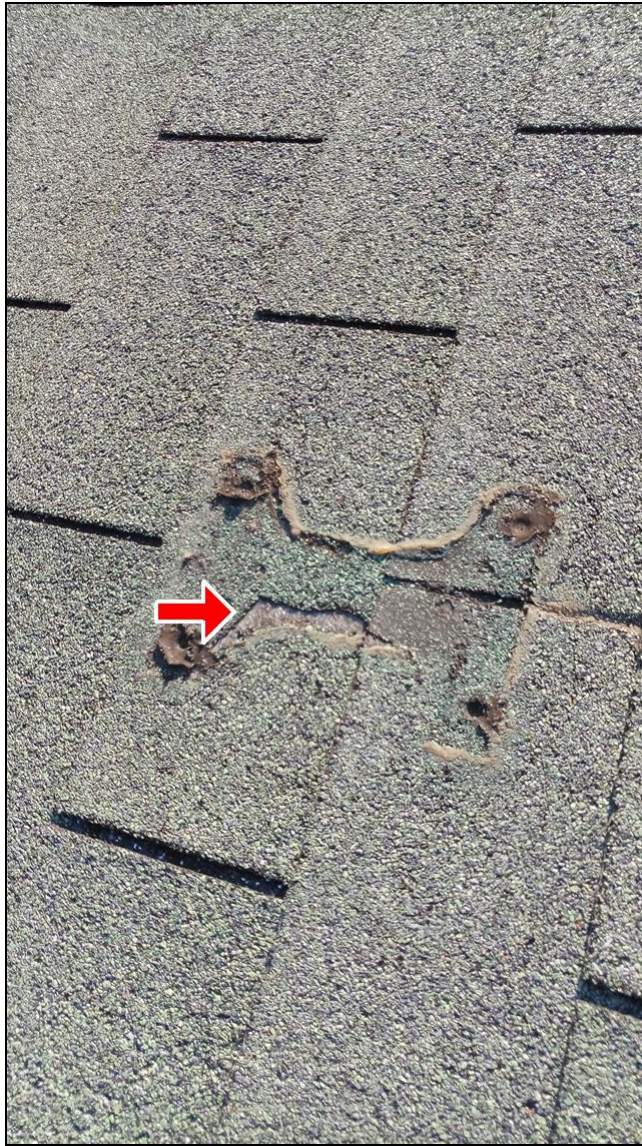
1.0 Item 5(Picture) Damaged shingles
