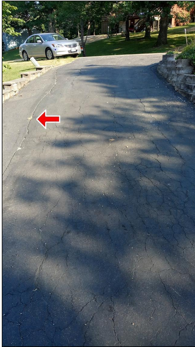
2.4 Item 6(Picture) Stress crack parallel to retaining wal
