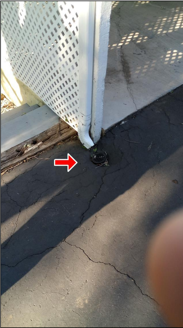
1.3 Item 1(Picture) This drain likely overflows
