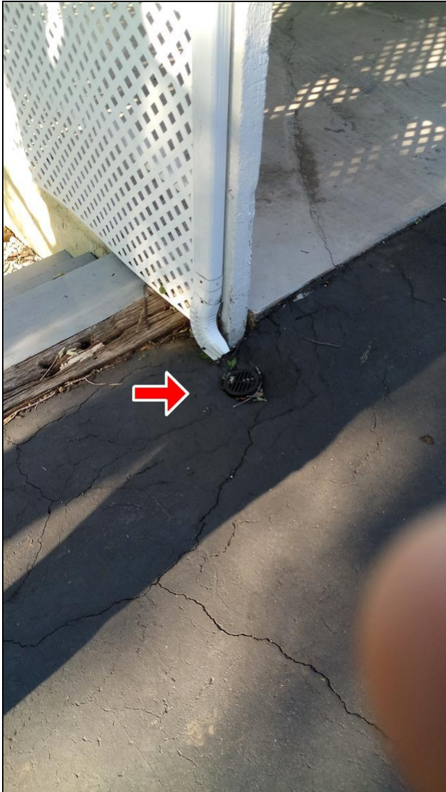
1.3 Item 1(Picture) This drain likely overflows
