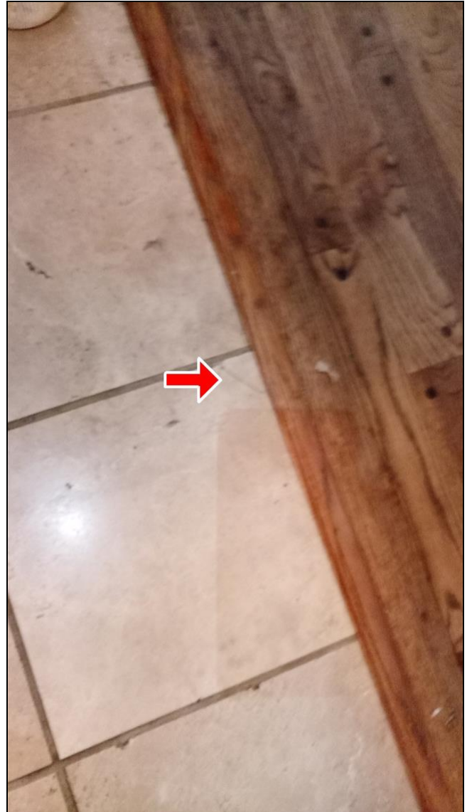
8.2 Item 2(Picture) Tile cracked
