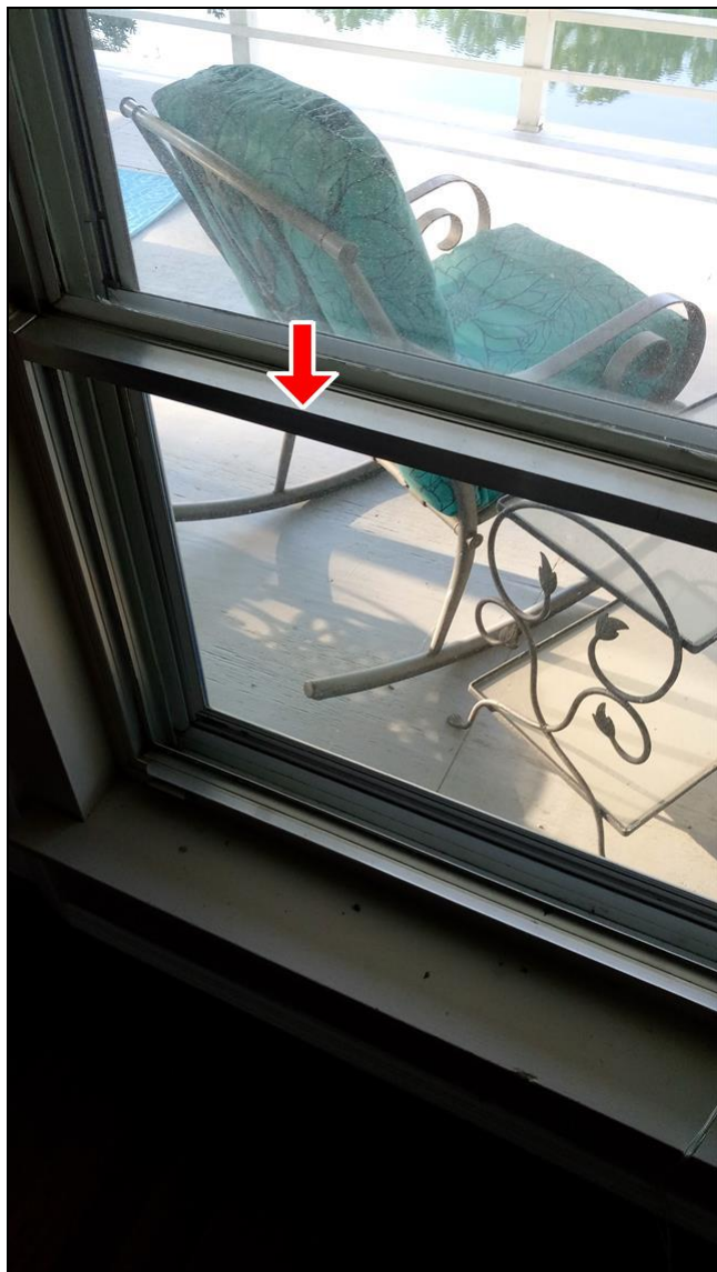
8.6 Item 1(Picture) Missing pane of glass
