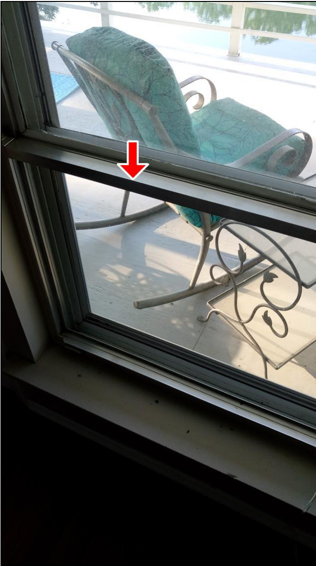
8.6 Item 1(Picture) Missing pane of glass
