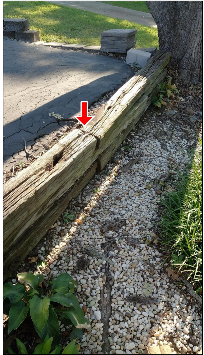
2.4 Item 4(Picture) Retaining wall failed
