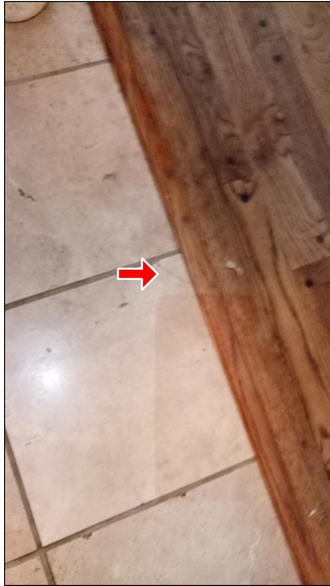
8.2 Item 2(Picture) Tile cracked
