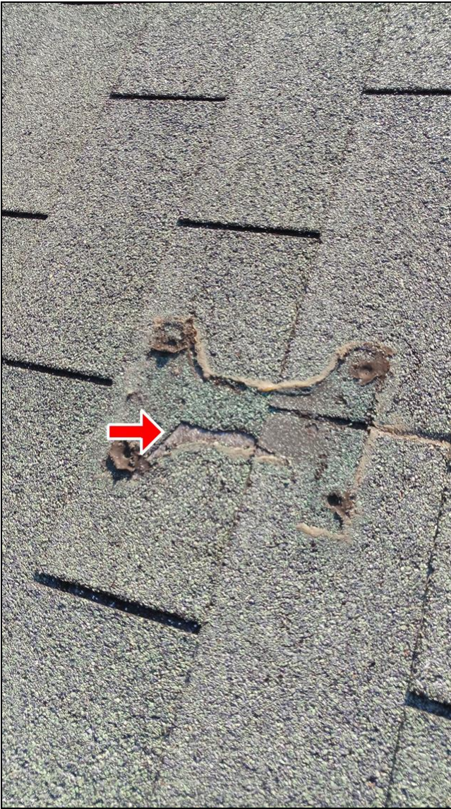
1.0 Item 5(Picture) Damaged shingles
