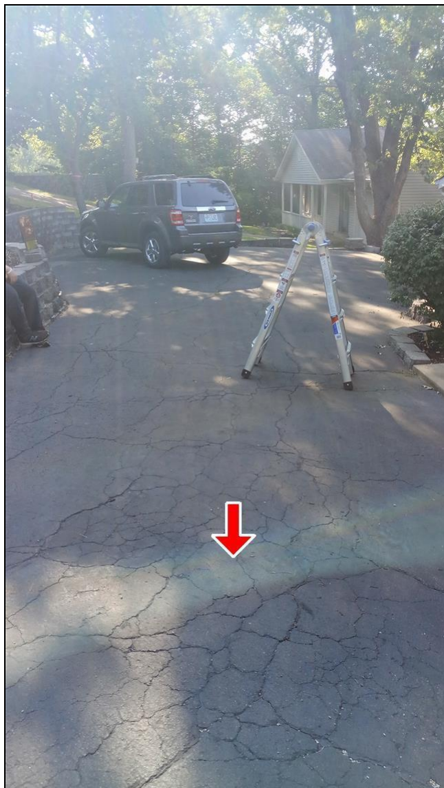
2.4 Item 7(Picture) Normal alligator cracking
