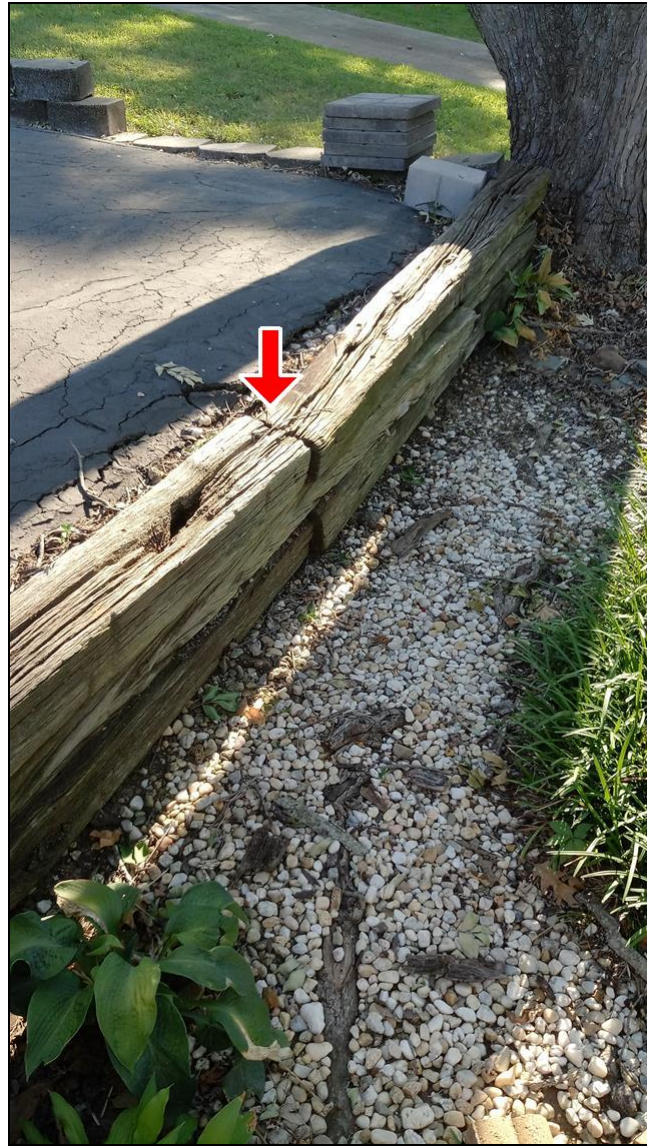
2.4 Item 4(Picture) Retaining wall failed
