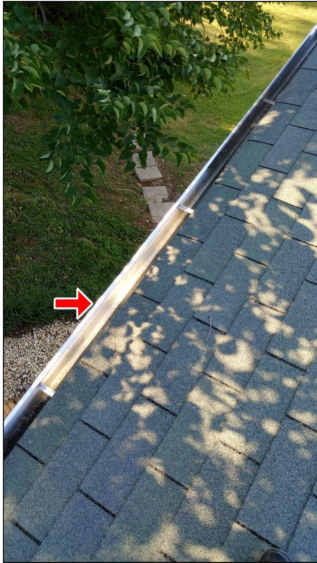
1.3 Item 2(Picture) Missing gutter guard
