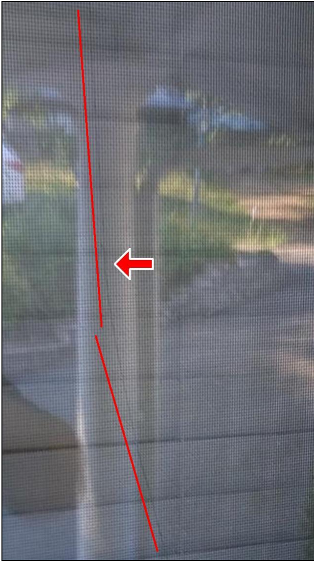
2.2 Item 1(Picture) Cracked front facing window
