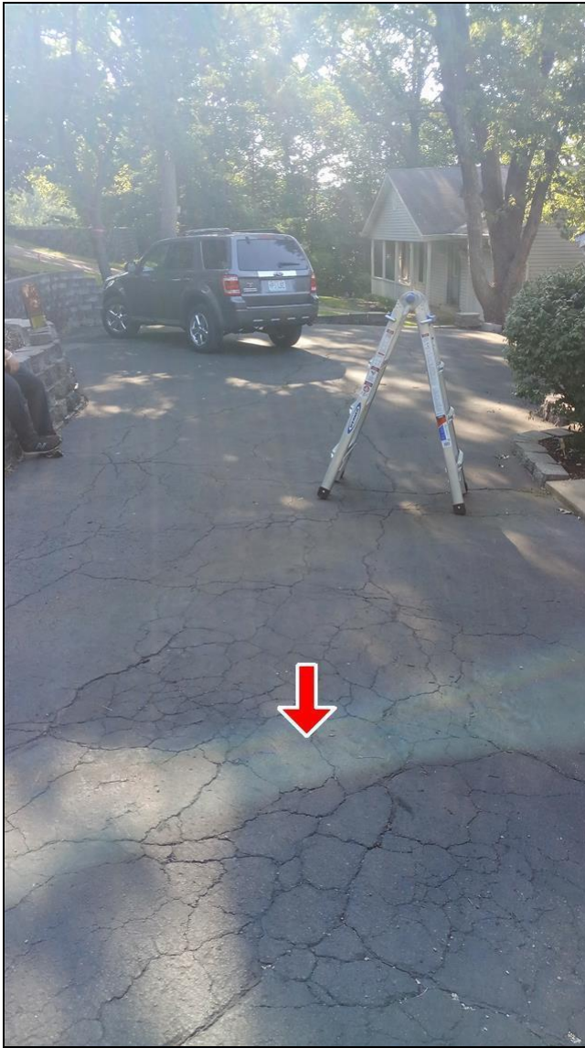
2.4 Item 7(Picture) Normal alligator cracking
