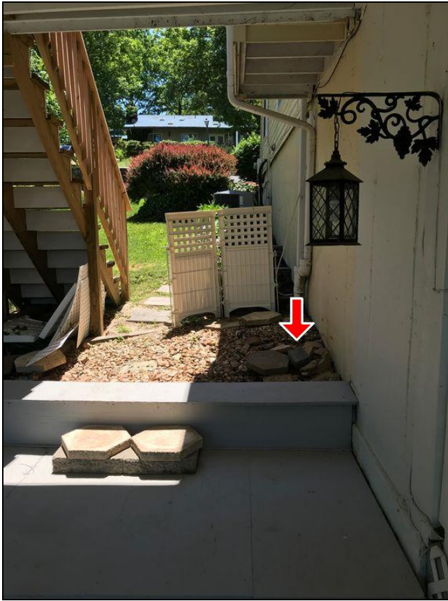
1.3 Item 3(Picture) Area drain likely overflows
