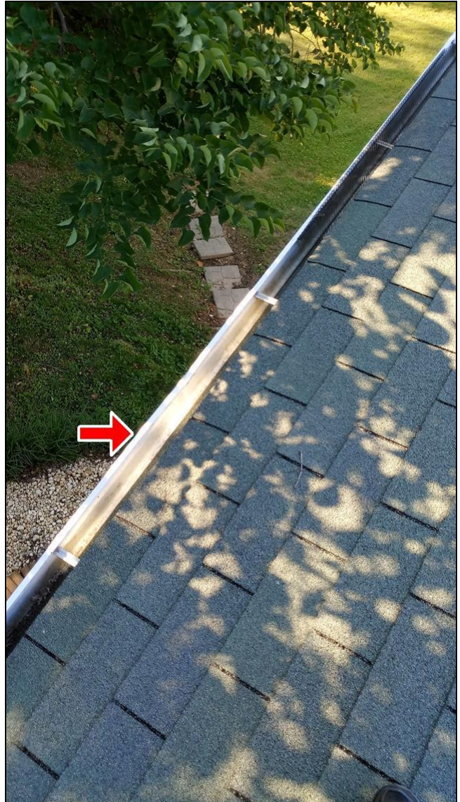
1.3 Item 2(Picture) Missing gutter guard
