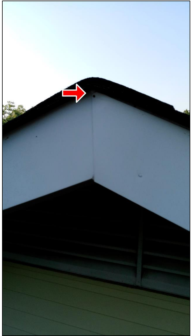
1.0 Item 2(Picture) Missing ridge vent
